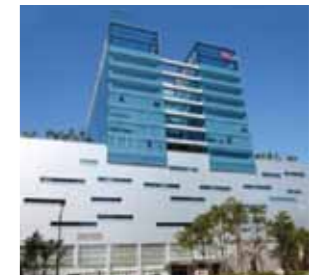
Gasan Data Center
