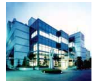
Incheon Data Center
